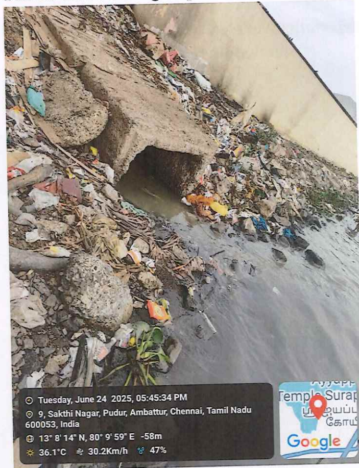
P1. Discharge of Sewage from storm water drain into Puzhal lake in Sakthi Nagar
