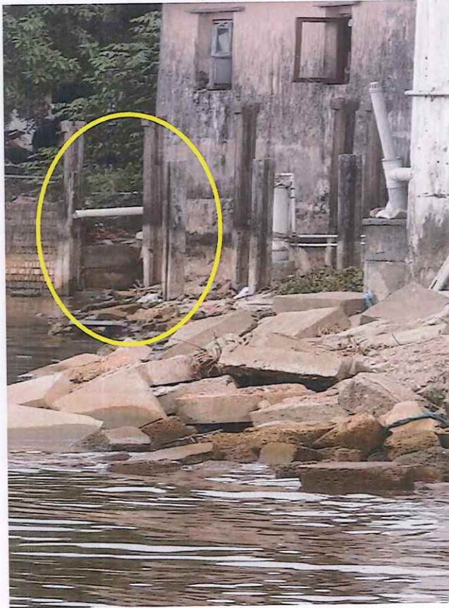
P3 – Sewage outlet from household in West Balaji Nagar, Kallikuppam directly discharging into Puzhal lake
